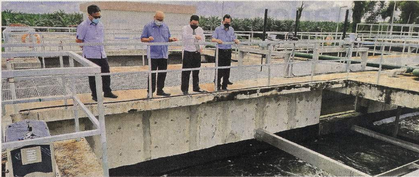
(From right) Lee, Lau, Miri mayor Adam Yii, as well as MCC secretary Morshidi Frederick check the sewerage system's aerated grit and grease chamber.
